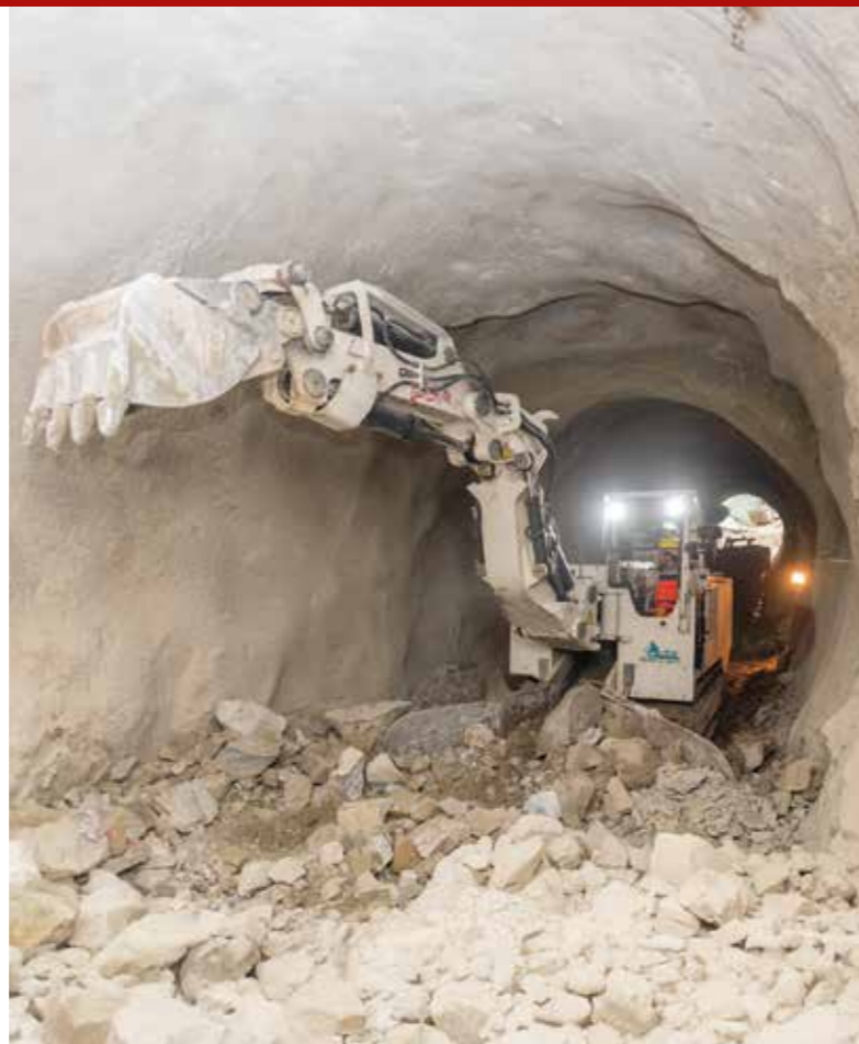
Tunnel loading machines
