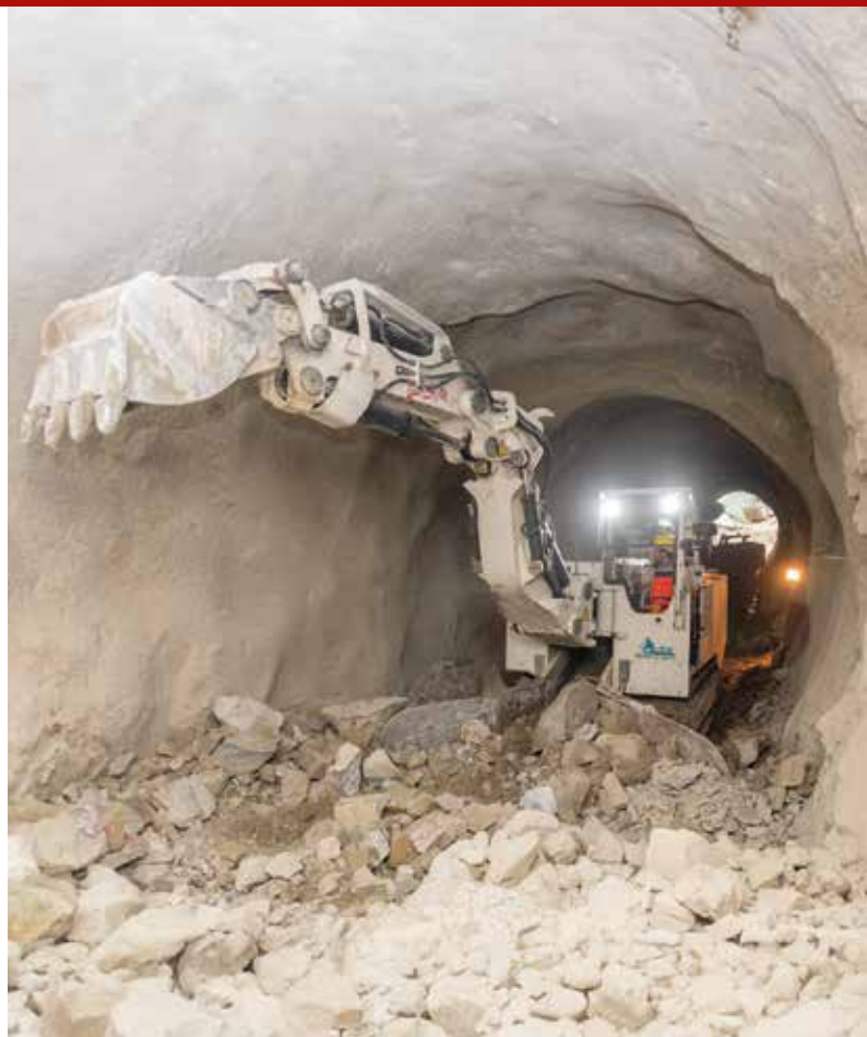
Tunnel loading machines
